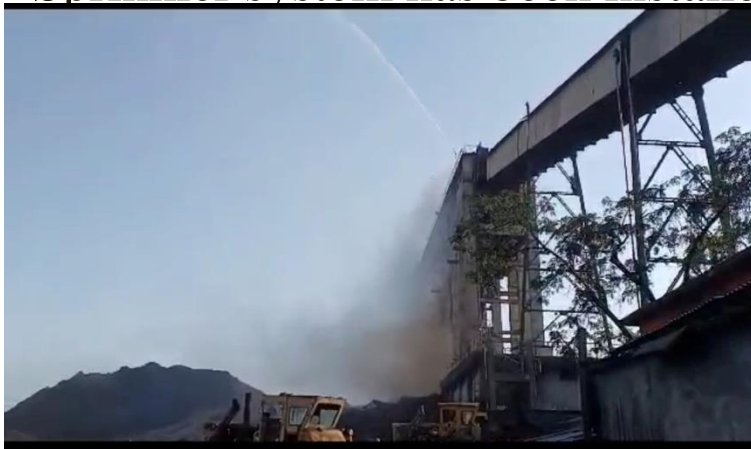
Sprinkler system installed in CHP
